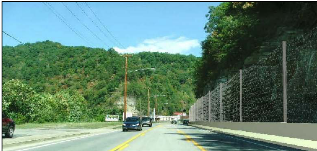
Alternative A - Rockfall Barrier
